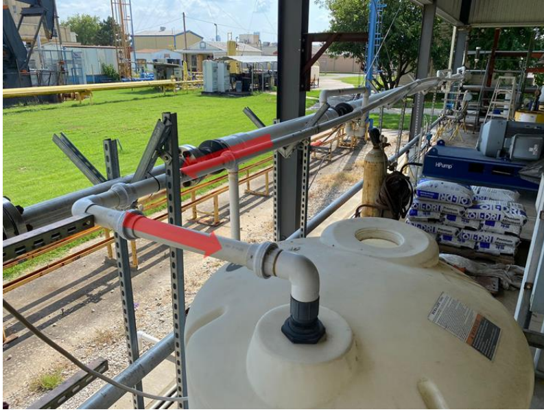
Figure A.10 Pipe-in-Pipe Heat Exchanger
