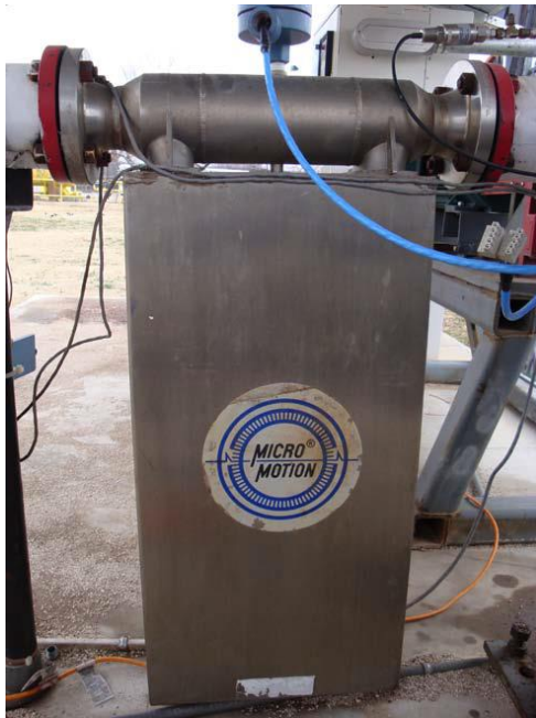
Figure A.7 Mass flowmeter
