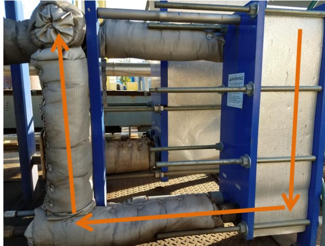
Figure 2.23 Flow path through heat exchanger
